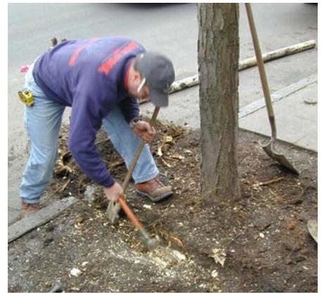
If you don't have room to go around tree roots, you can "shave" the roots with a hatchet by removing small roots and notching large ones about 3 inches below ground level to allow room for a new sidewalk over the roots.
