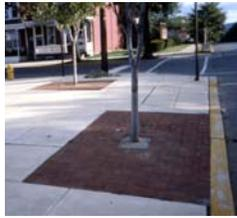
If you are installing a new sidewalk, you can go around a tree, or create a large tree pit covered with bricks that can be removed as the tree grows.
